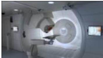
360°GRANTRY TREATMENT ROOM
