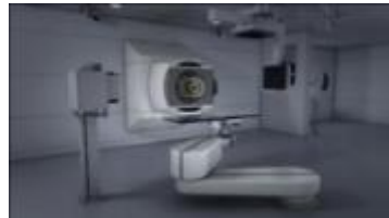
FIXED BEAM TREATMENT ROOM
